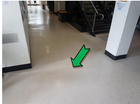
Photo 4. Interior, ground level, northern elevation, throughout, floor – suspected non asbestos-containing sheet vinyl.
