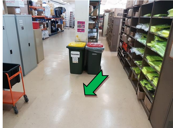
Photo 2. Interior, ground level, throughout, floor – non asbestos-containing vinyl floor tiles.
