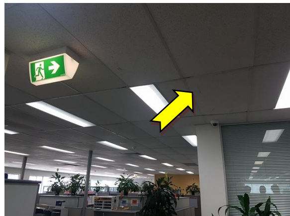
Photo 6. Interior, level 1, northern elevation, throughout, ceiling – suspected SMF-containing compressed ceiling tiles.
