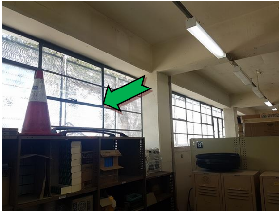
Photo 3. Interior, ground level, throughout, window frames – non asbestos-containing caulking.
